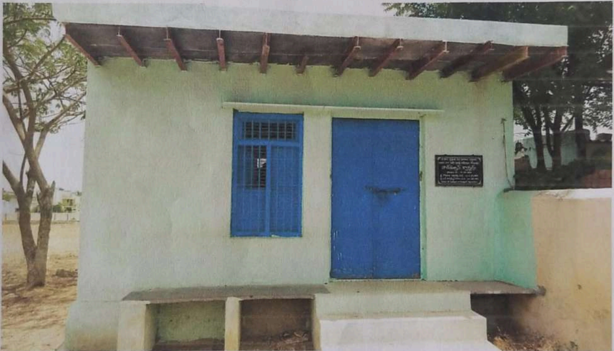
After Construction Watchmen Quater
